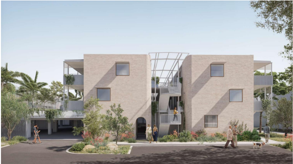
Figure 2: Image from Gallagher Street to buildings S5B-A and S5B-F (Easy Block).
